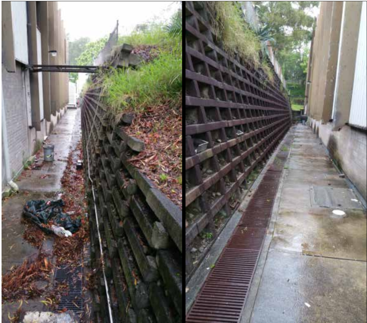
Figure 3: Existing Crib Retaining Wall along Eastern edge of existing NBN building (looking north, looking south)
